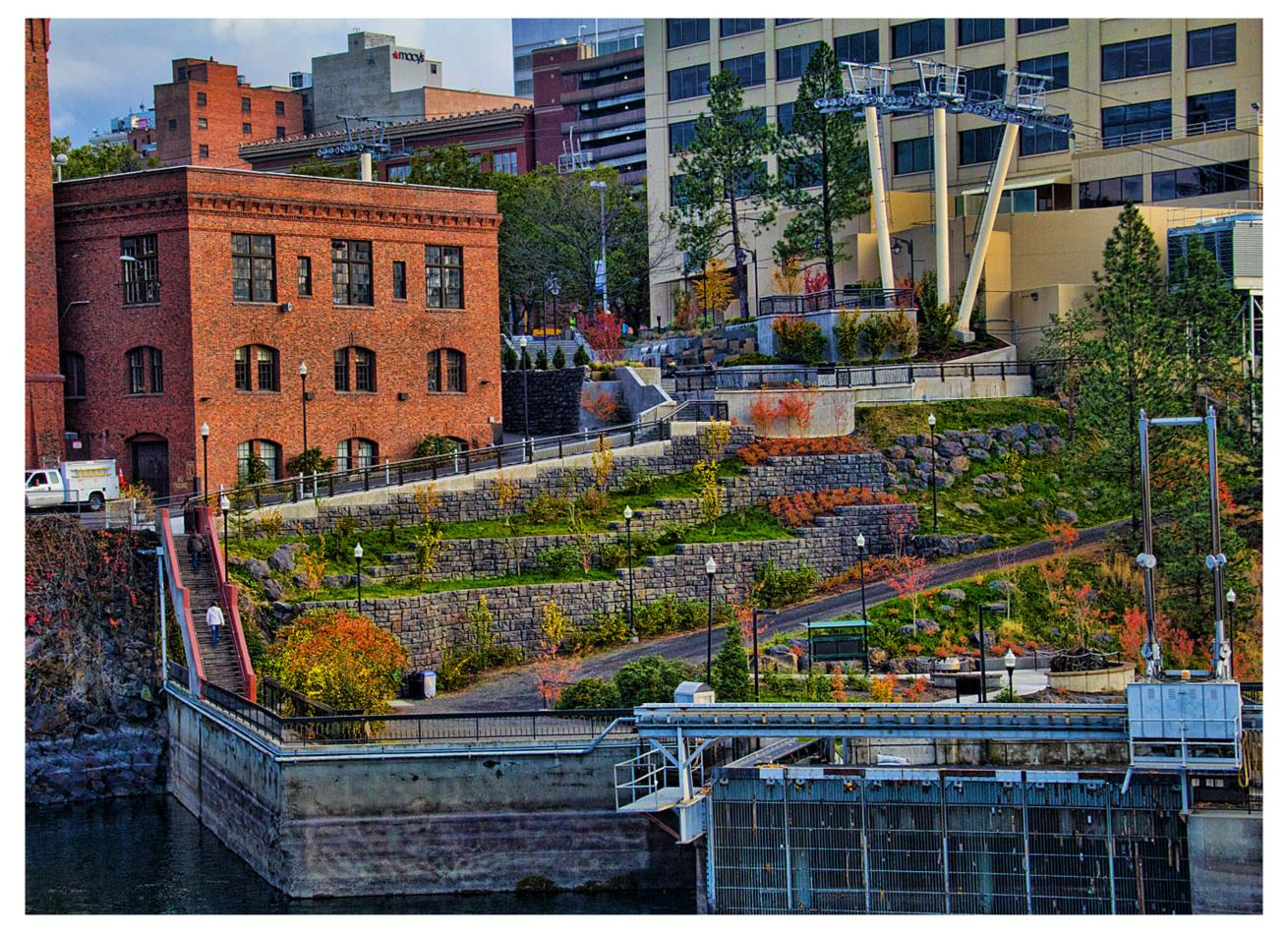
TOPOGRAPHY - Extreme grade changes presented a design challenge. Concrete walls and prefabricated concrete blocks were utilized for a terracing solution. Stained to reflect basalt rock, and planted with natives, naturalize the appearance. (Intake structure in foreground).
